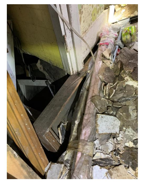
Kitchen has collapsed into basement and little to no floor remains (refrigerator has fallen into the basement)
